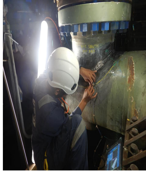
YEAR : 2023 PROJECT : PIPING PAUT LOCATION/REGION : BATAM,INDONESIA
