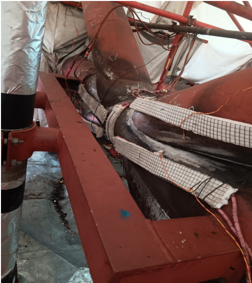
YEAR : 2024 PROJECT : PRE HEATING ON CHORDS AND BRACING LOCATION/REGION : SINGAPORE
