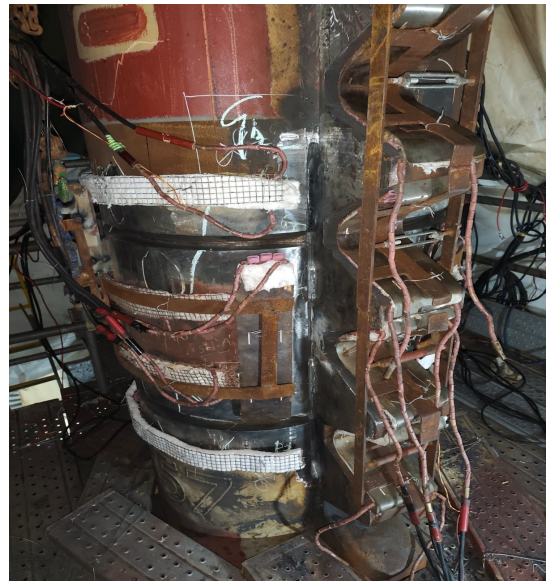
YEAR : 2024 PROJECT : PRE HEATING ON JACKUP LEG'S GEARS LOCATION/REGION : SINGAPORE
