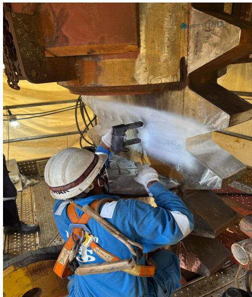
YEAR : 2025 PROJECT : MPI ON JACKED LEG – WTIV PROJECT LOCATION/REGION : SINGAPORE
