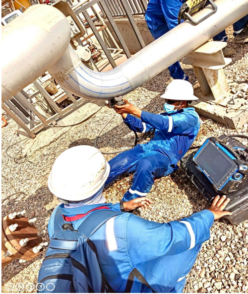
YEAR : 2021 PROJECT : PIPING PAUT LOCATION/REGION : BATAM,INDONESIA
