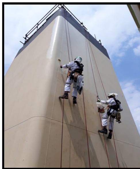
YEAR : 2018 PROJECT : ROPE ACCESS MAINTANANCE JOB ON HULL LOCATION/REGION : INDONESIA
